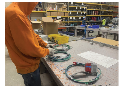
Room in a box assembly fabrication.
