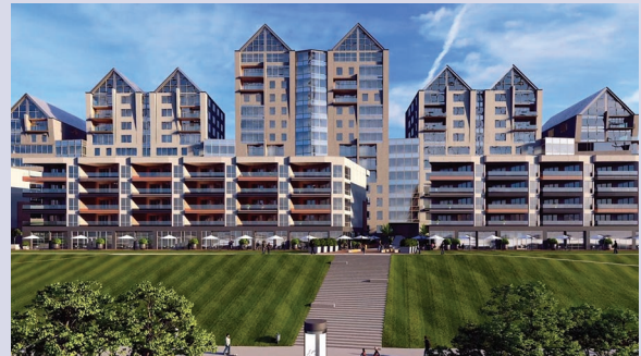
The Ovation project.
